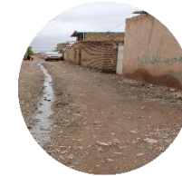
Moisture penetration problems
