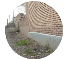
Using Waterproofing sheets At the base of the wall
