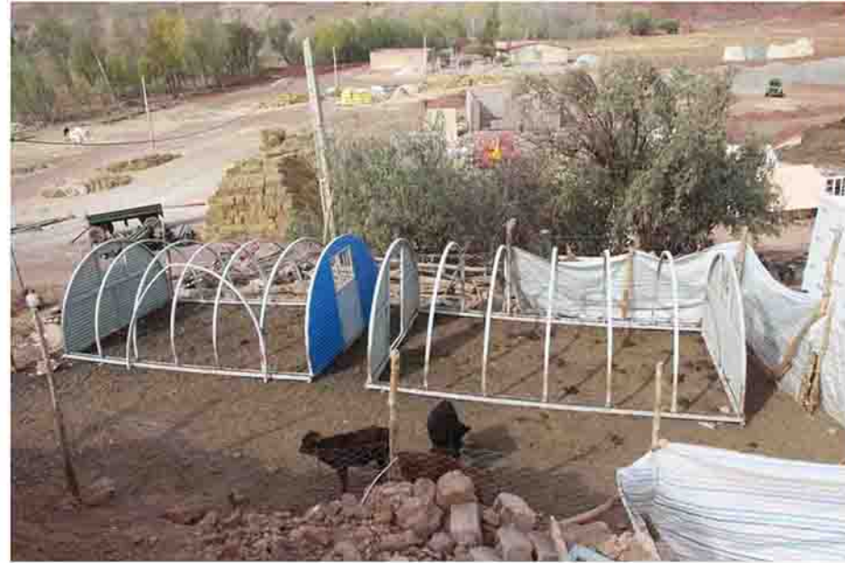
- The unfinished conexas for ranching,unused and abandoned .
